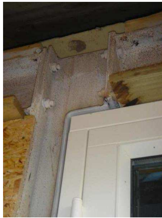
When a Support Column Clashes with a Window
