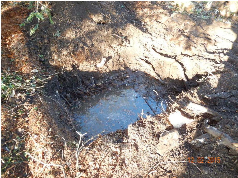
Surface Water Soakaway Tests to BRE 365.
