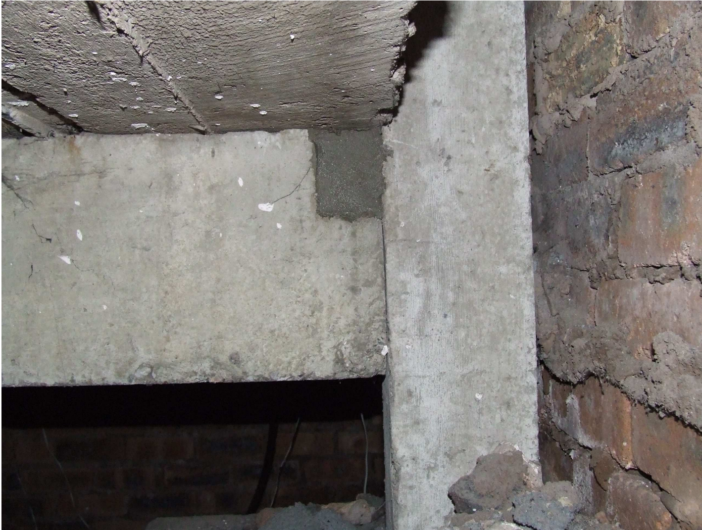
Whitson Fairhurst - Infilled Pin Joint between Floor Beam and Column.
